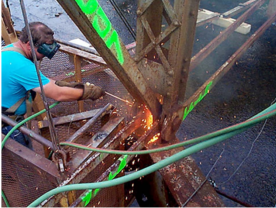
Figure 27. Piercing Center of Pin
