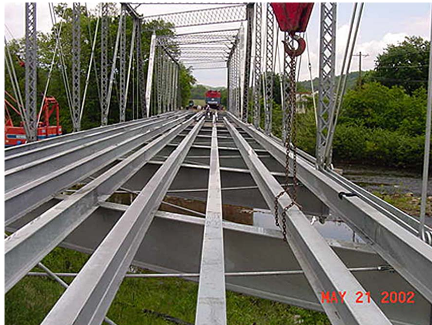
Figure 34. Installation of Stringers
