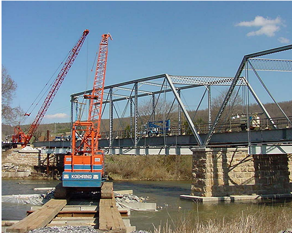
Figure 21. Crane Locations During Re-erection of Trusses
